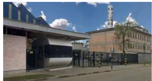
Macom Headquarters Plant (Guarulhos, Brazil)
