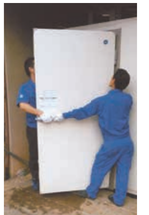
Product repair work
